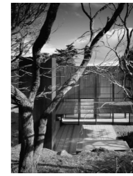
PENINSULA HOUSE Location: Victoria, Australia Design: 2000 - 2001 Construction: 2001 - 2002
